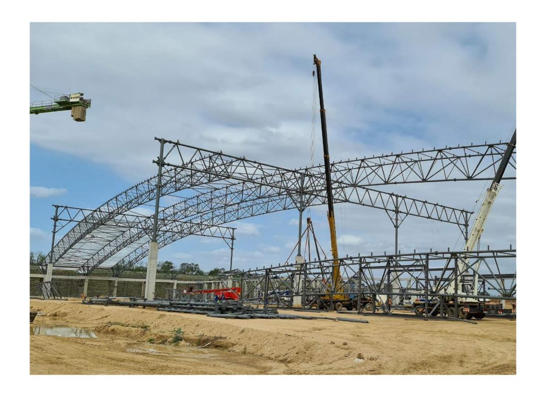
The two roof gables structure provided support to approximately 2200m2 of side wall gable cladding at each end. Two dimensional tubular pipe trusses were used to support the up to 16m high gable ends. The steelwork roof was designed to support a 200mm thick insulated roof covering as well as making allowance for future solar power panels configuration.
