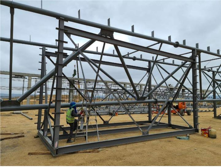
A major concern throughout the installation phase of the Project was that the holding down bolts at the two concrete abutments of the roof would talk to each other such that 210 meters of roof truss would fit snugly between the steel buttress frames once they were mounted on them.
