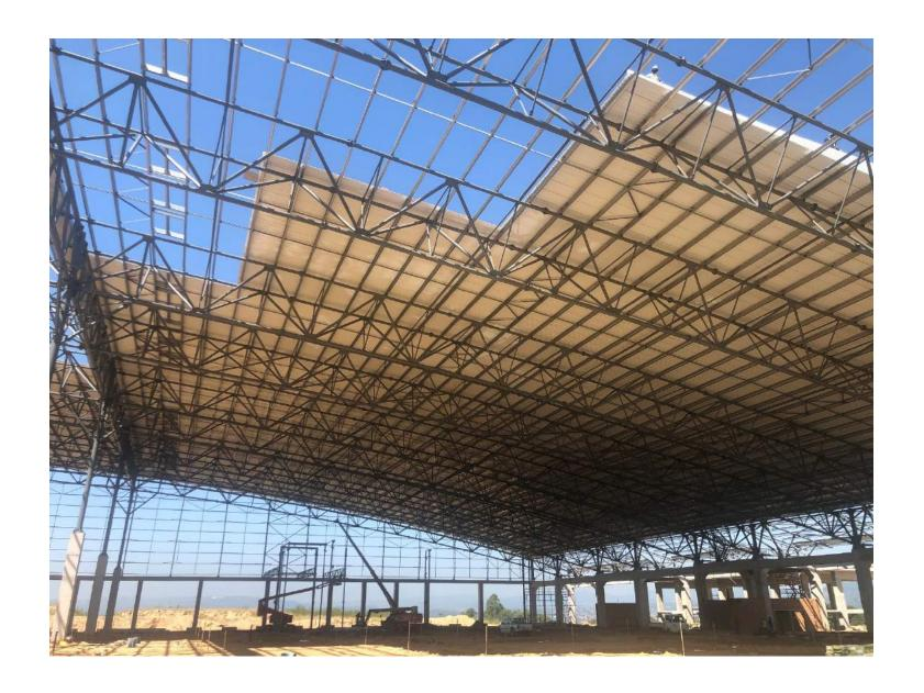
The Widedek ceiling sheets were installed in various lengths lapped over the purlins since they do not form part of the weather envelope.
