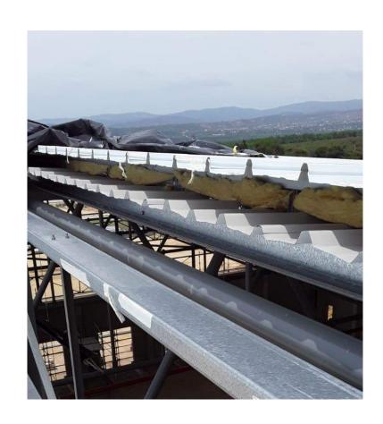
The roof is split into three equal segments for sheeting separated by gutters with the 68m long SAFLOK roof sheets being rolled on site and pushed up a scaffold ramp onto the roof.
