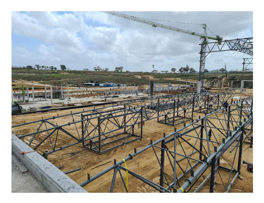
Assembly of the toblerone trusses on the site necessitated the provision of a number of assembly frames which had to be set out, lined and levelled to ensure the accurate assembly of each truss before hoisting.
