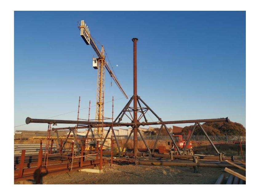
Similarly the configuration of the support column / girder / truss intersection was incredibly complicated and the trial assembly of this section of the roof at the workshop was seen as being critical to the success of the Project.
