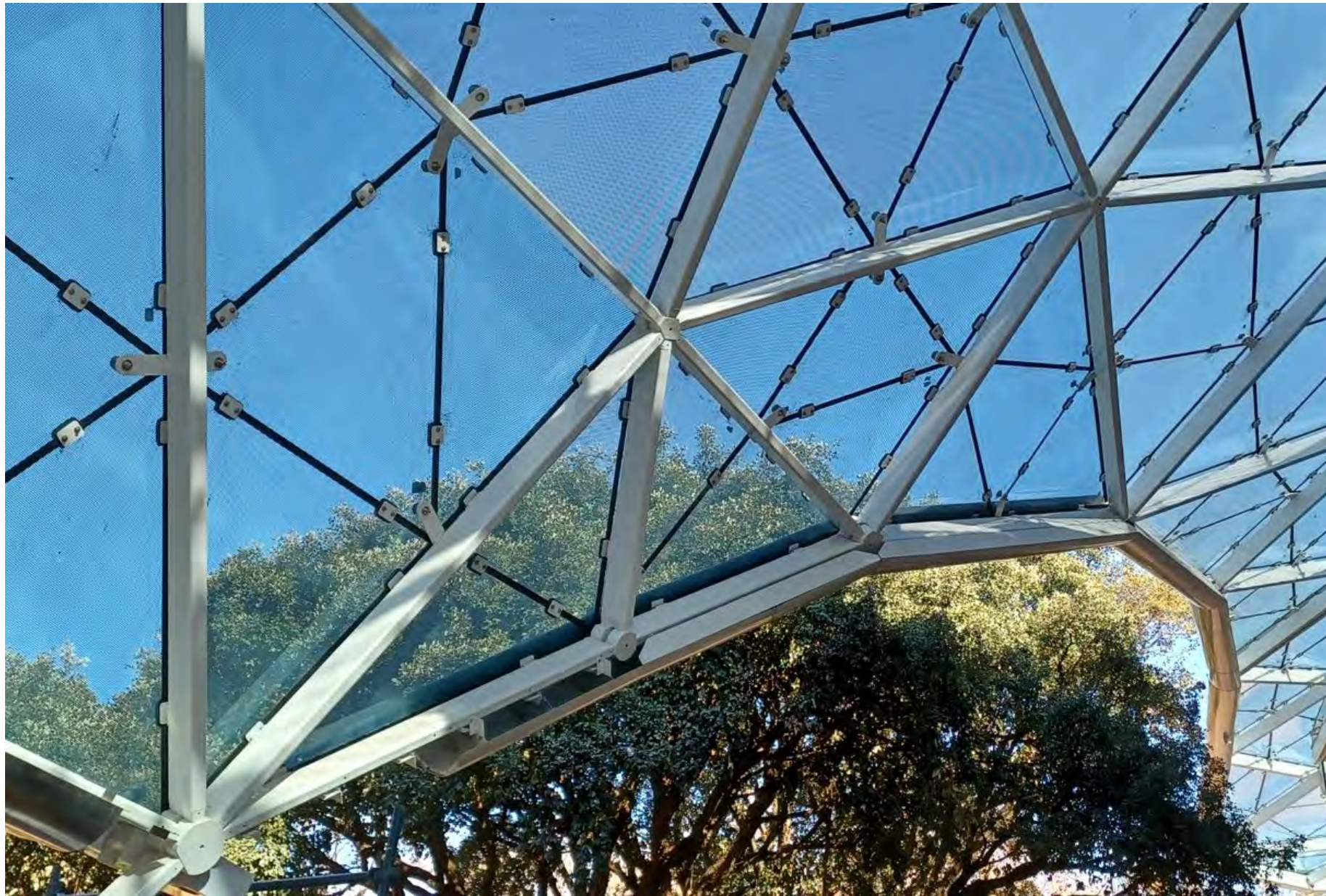
Bull Nose Wrapping Around the Structure
