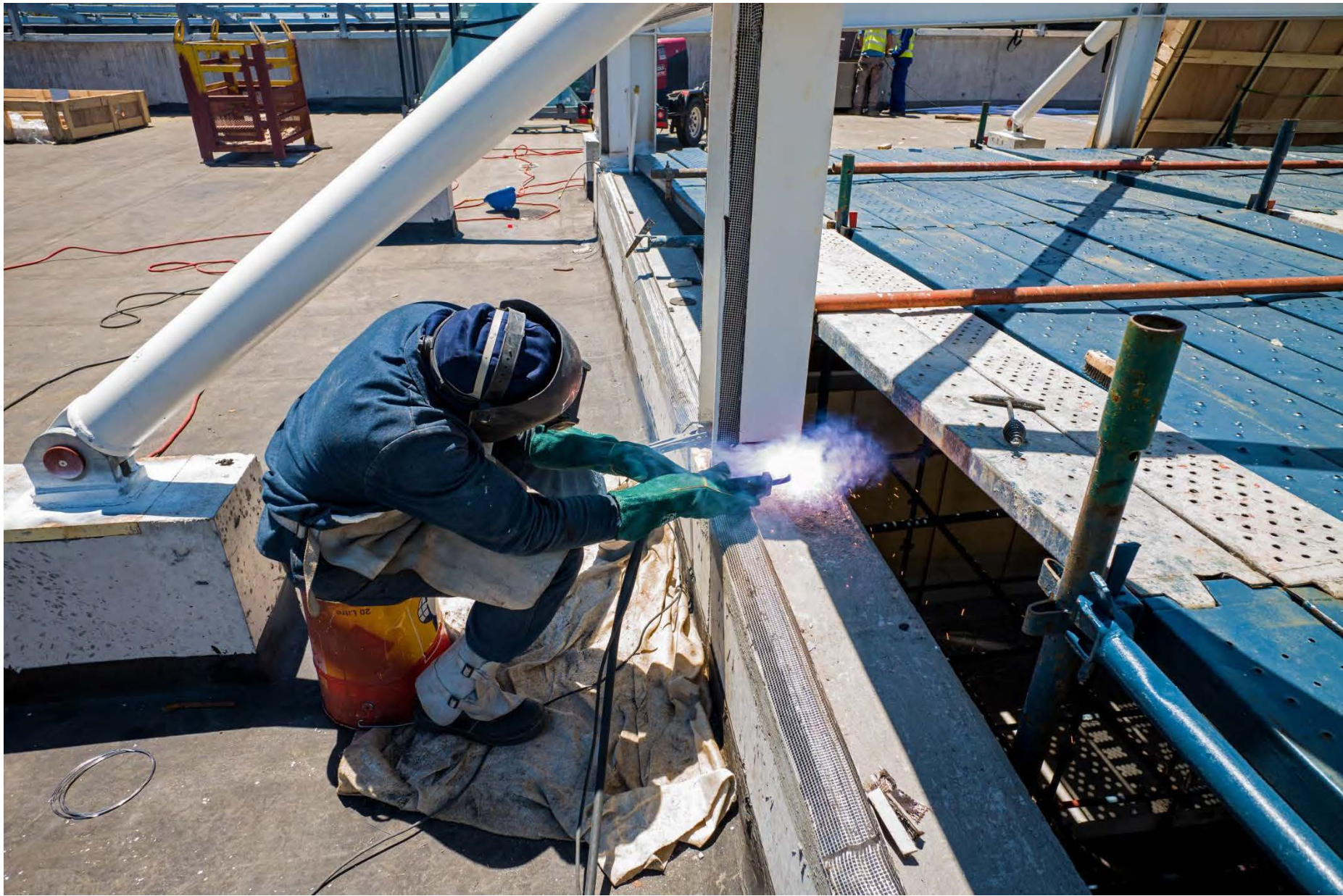
Atrium Steelwork Installation
