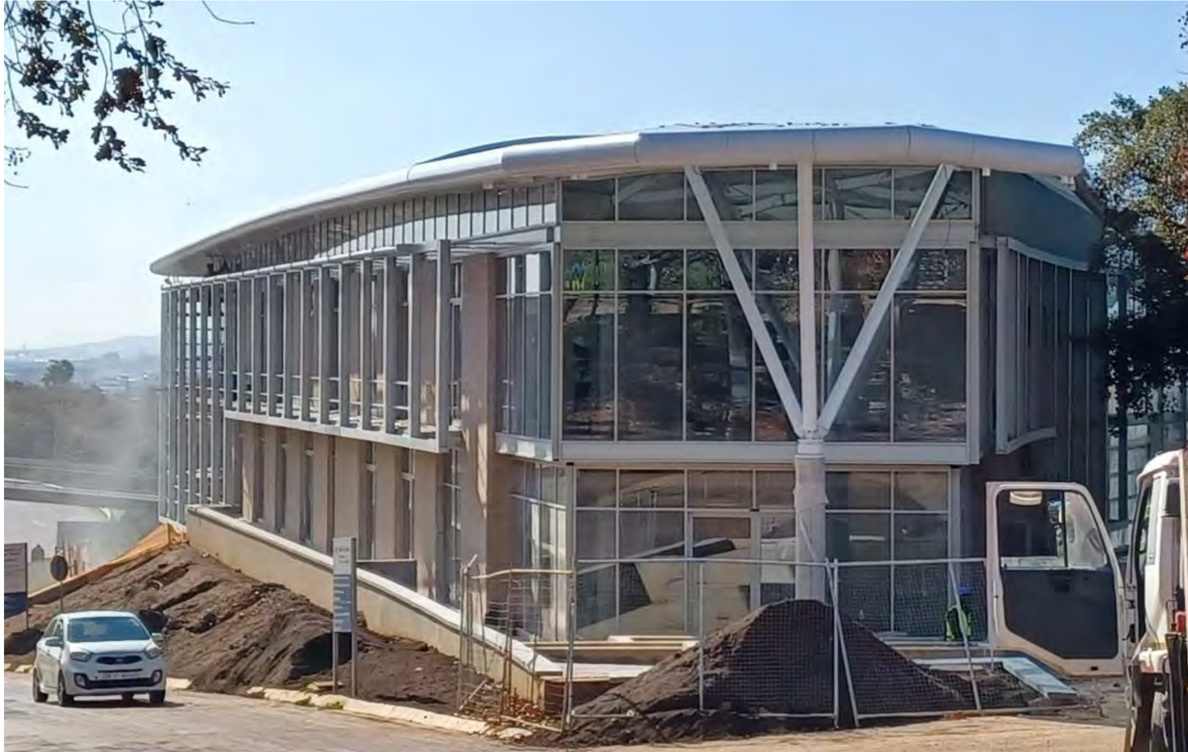
Bull Nose Wrapping Around the Structure
