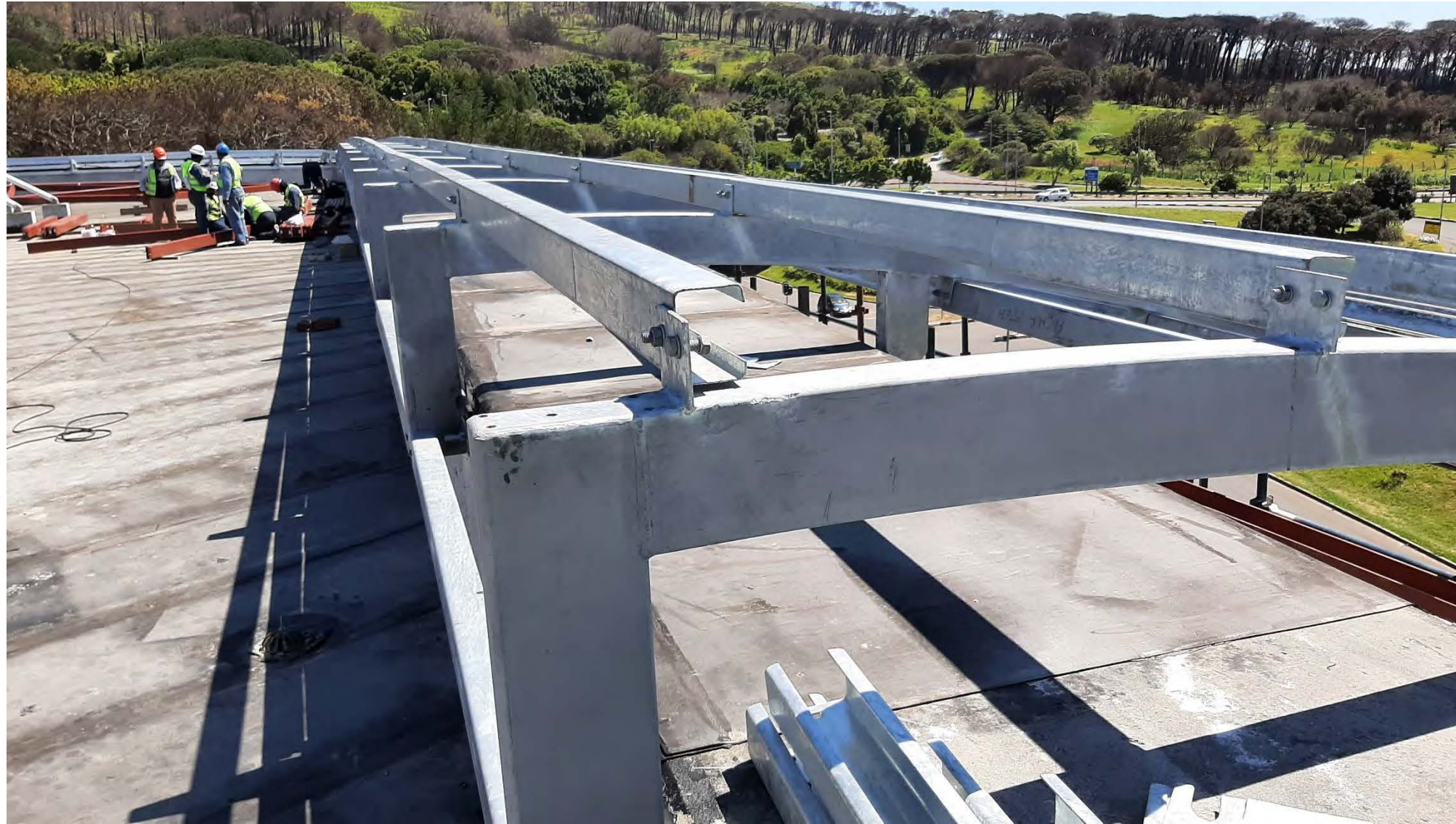
Eyebrow Steelwork Installation
