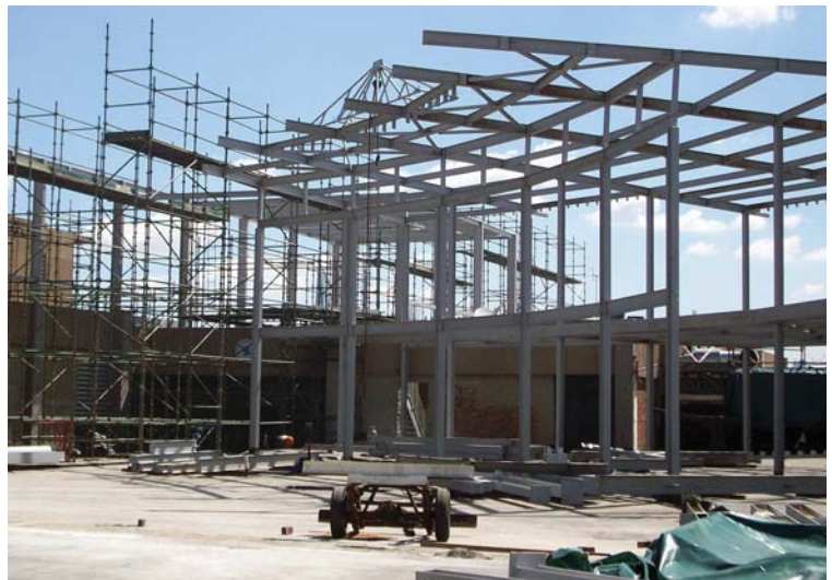
Primary steel frame being erected prior to fixing of lightweight steel.
