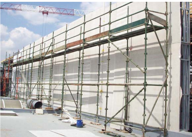
Cladding of lightweight steel frame wall.
