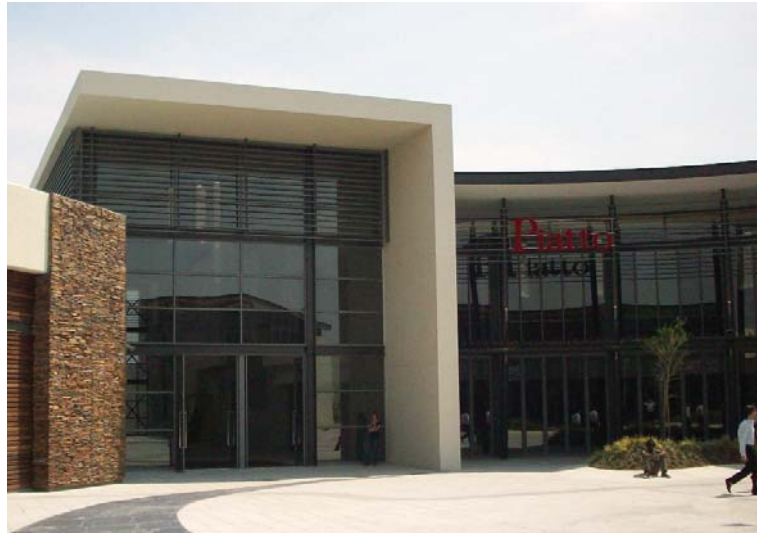
10m high entrance wall and canopy constructed with lightweight steel.
