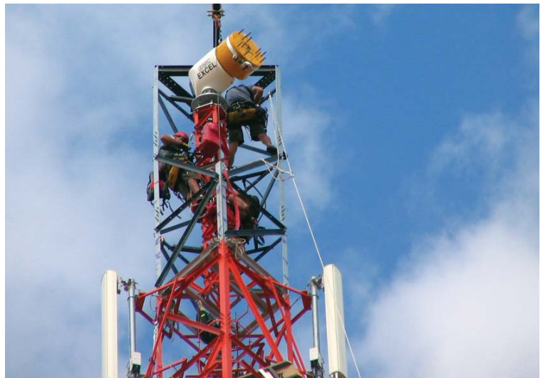
The attachment of the turbine at the top of the tower. The temporary structure also helped the workers by providing a perch from which to work.
