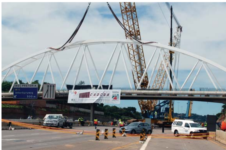
The impact on traffic is minimised with the erection of a steel bridge over operational roads.
