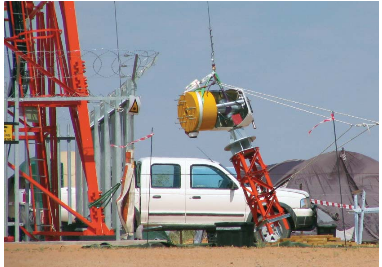
The turbine with the top section of the mounting structure at the start of the lift.
