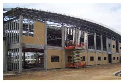
Light Frame Homes (Cape Town) supplied and cladded the light steel frames of the Novo warehouse.
