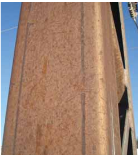
One of the first big projects using 3CR12 was the railway electrification masts in Port Elizabeth, which went into service in 1982, and are still operating, at zero maintenance cost, some 30+ years later.
