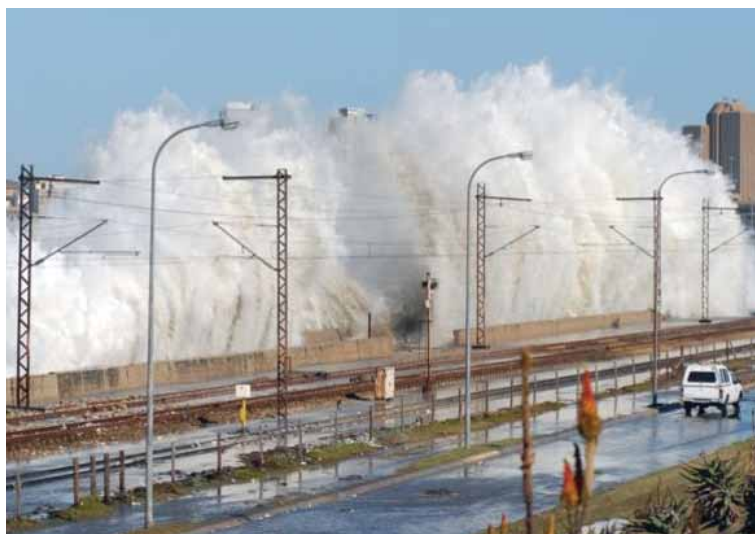
One of the first big projects using 3CR12 was the railway electrification masts in Port Elizabeth, which went into service in 1982, and are still operating, at zero maintenance cost, some 30+ years later.
