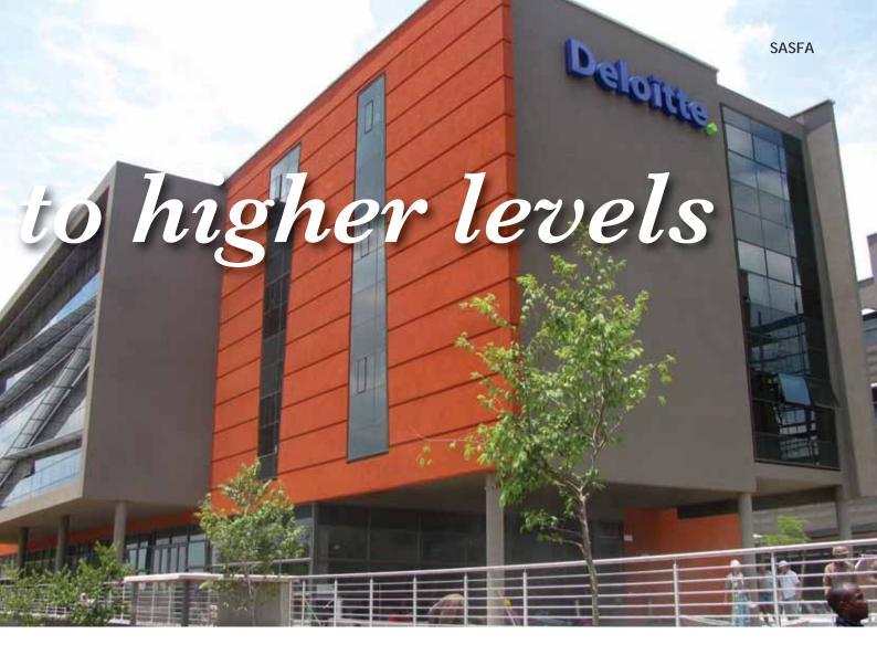
fixed. The external finish of the EPS consists of two layers of a special colour impregnated polymeric plaster. A reinforcing fibreglass mesh is embedded in the coating. This cladding system is referred to as EIFS (external insulating and finishing system). The inside of the light steel frames is clad with fire-resistant gypsum board. Additional insulation can be installed in the wall cavity, if required.
