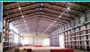
Warehouse Upgrade Kumba
