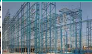
New Ferrochrome Furnaces Factory
