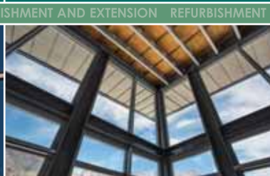
Roeland Park Office Block Development
