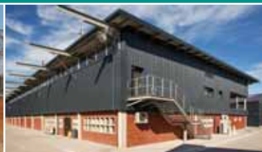
Ndabeni Electrical Depot
