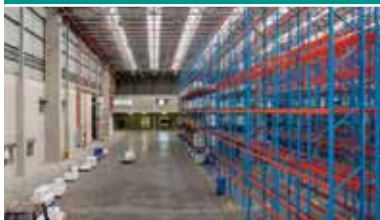
New Distribution Centre, Value Logistics
