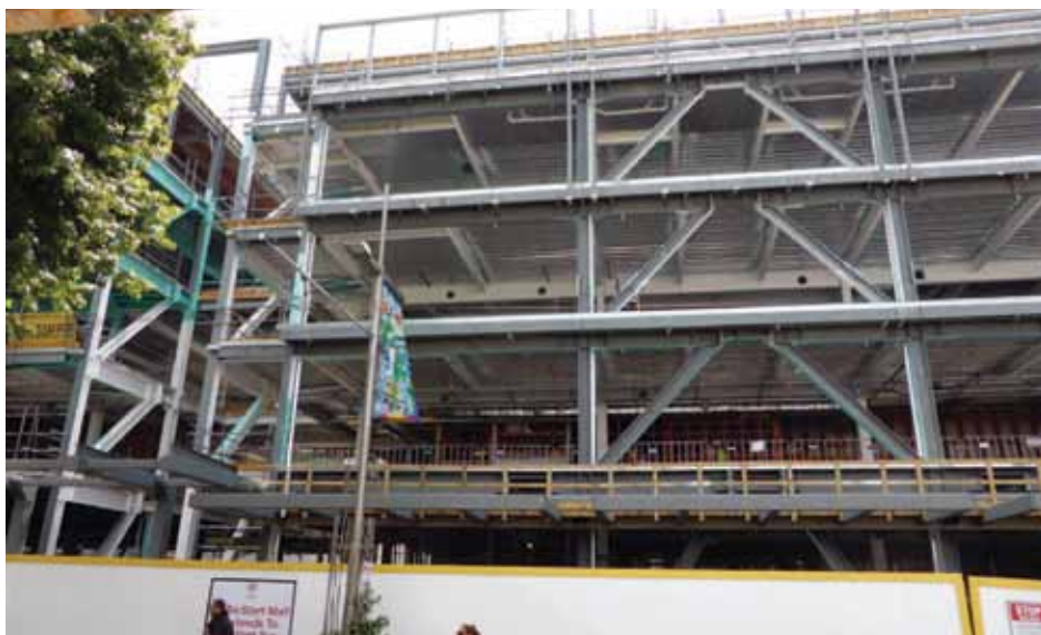
An EBF with replaceable links (left) and a close-up of a link in an inverted-V braced frame (right).
