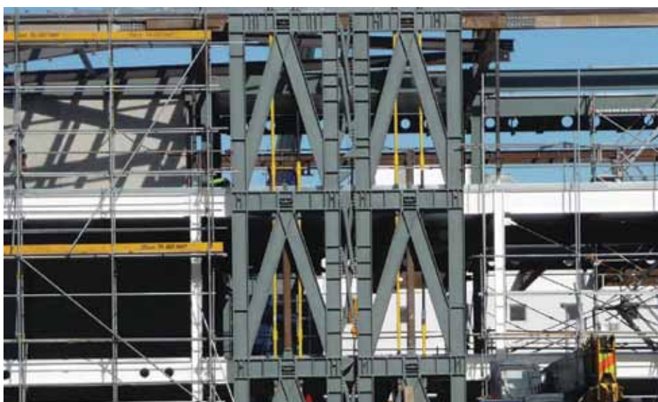
A rocking frame system with energy-dissipating couplers between the frames.
