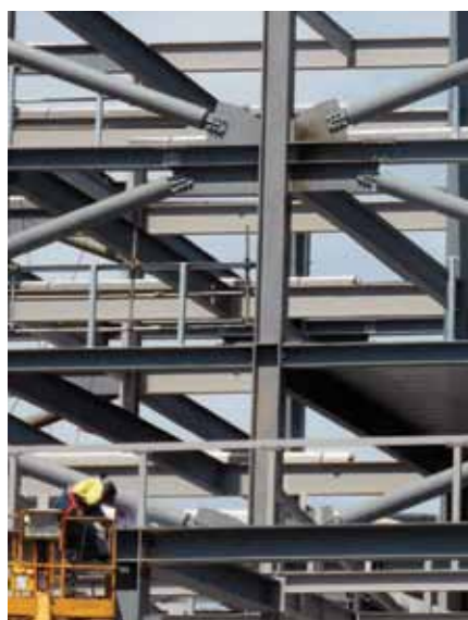
A BRB frame (left) and a column connection at mid-bay of the frame (right).
