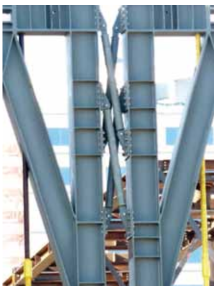
A rocking frame system with energy-dissipating couplers between the frames.
