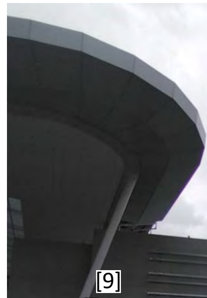
Fabrication of aluminium composite panels for exposed ceiling closure
